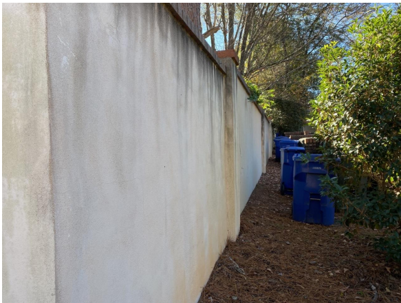
Block and stucco wall
