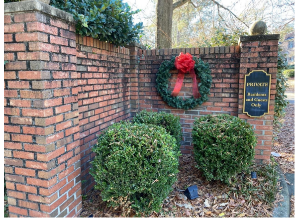
Brick and mortar wall
