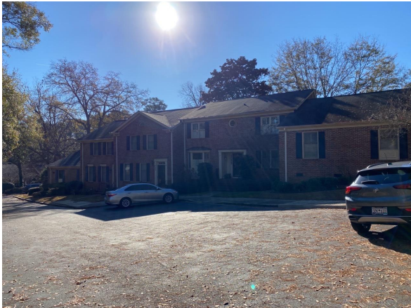
Asphalt parking area
