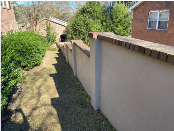
Block and stucco wall
