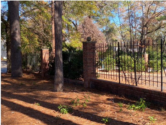
Iron perimeter fence
